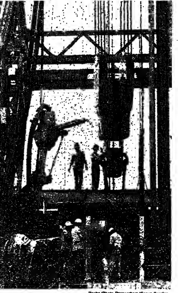
Drilling rig is mounted on a barge in the river. The Nigerian Government is now rigidly controlling oil wealth.
